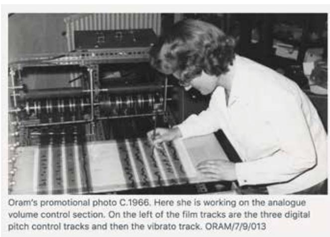
Oram's promotional photo c.1966. Here she is working on the analogue volume control section. On the left of the film tracks are the three digital pitch control tracks and then the vibrato track. ORAM/7/9/013
